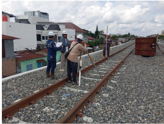
Figure 2. Elevation Ballast Data Collection and Thermite Welding Refinement
