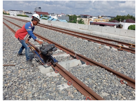
Figure 2. Elevation Ballast Data Collection and Thermite Welding Refinement
